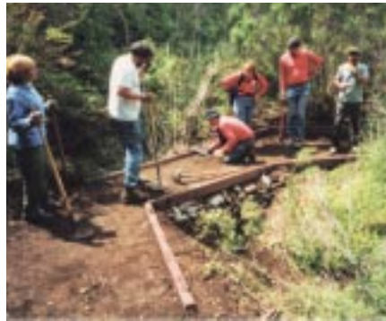
The big culvert on Acorn Trail
