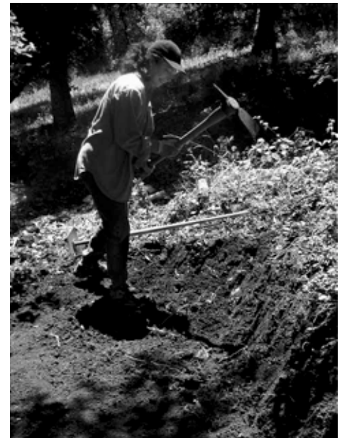
Working on one of the switchbacks at Arastradero
