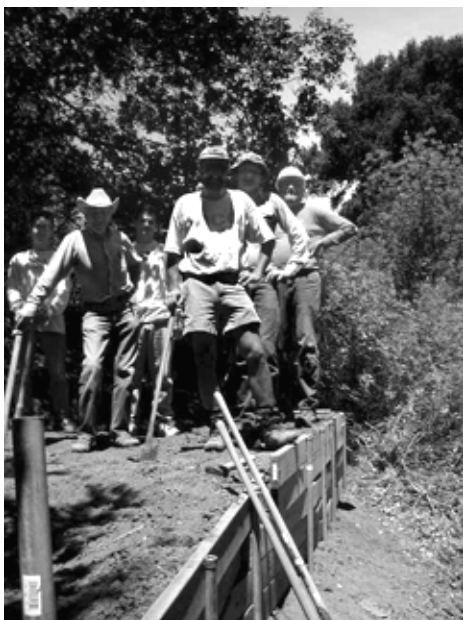
The retaining wall crew show off their hard work
